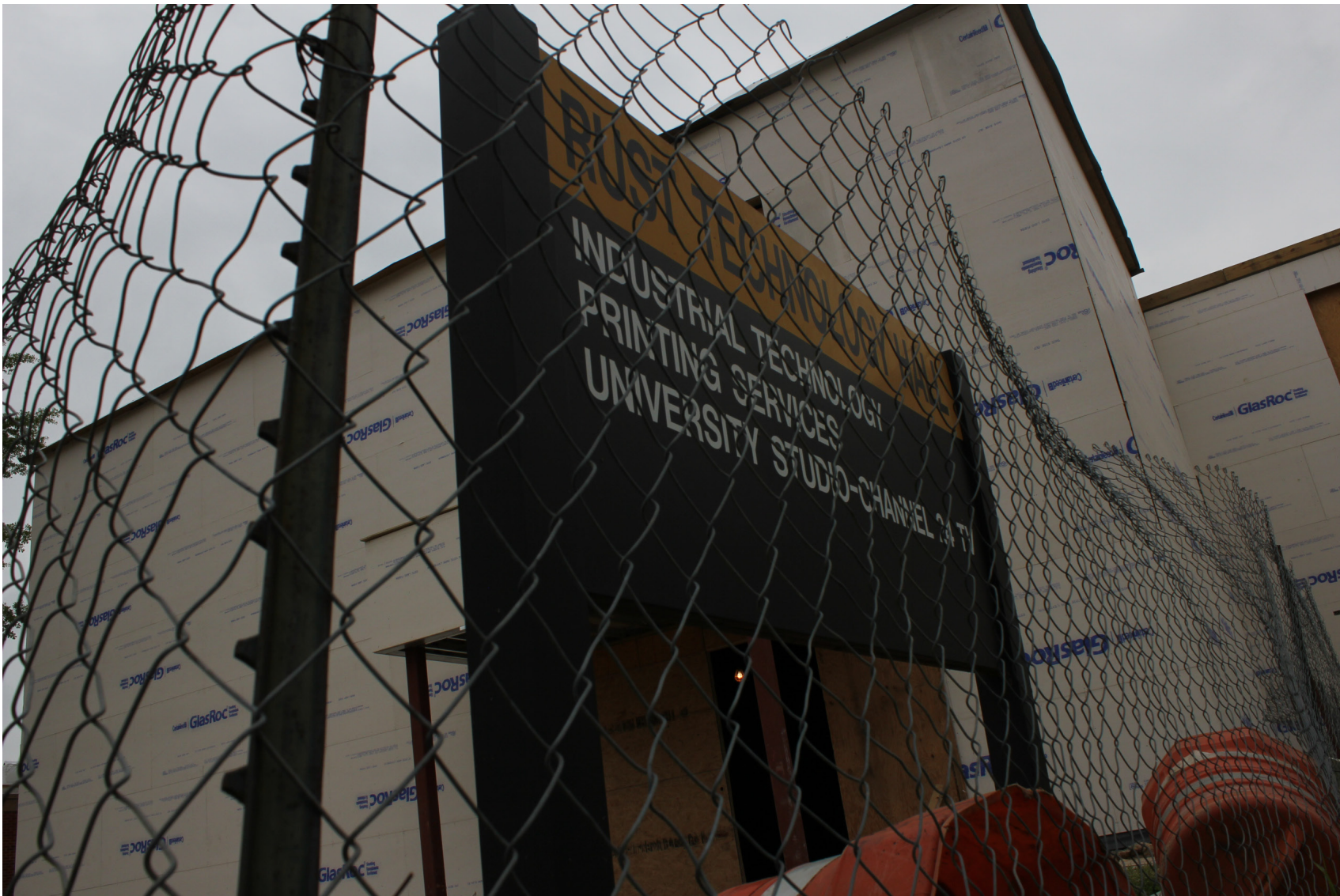
The present state of Rust Technology Hall.
